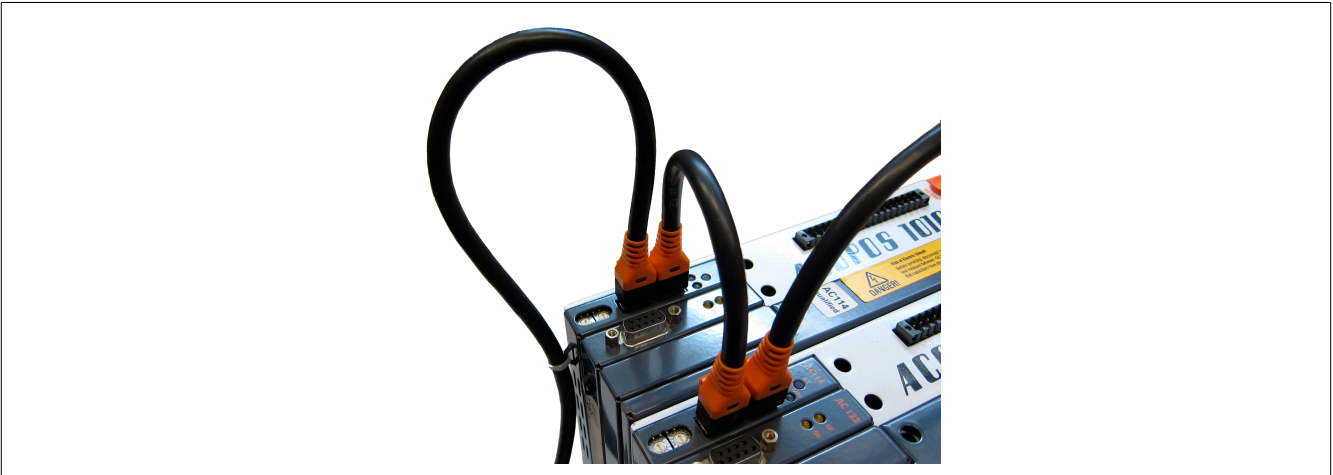
Figure 90: Connecting cables to plug-in modules
